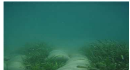
Sediment Tubes installed in propeller scars
